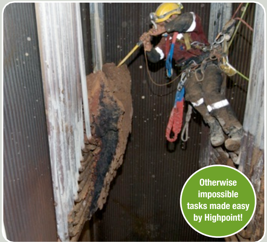
Above: Clinker removal from the platen superheater elements in a power station furnace.
